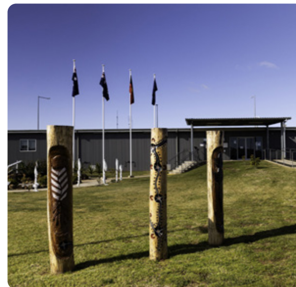
Macquarie Correctional Centre, Wellington. Photo courtesy of CSNSW.
